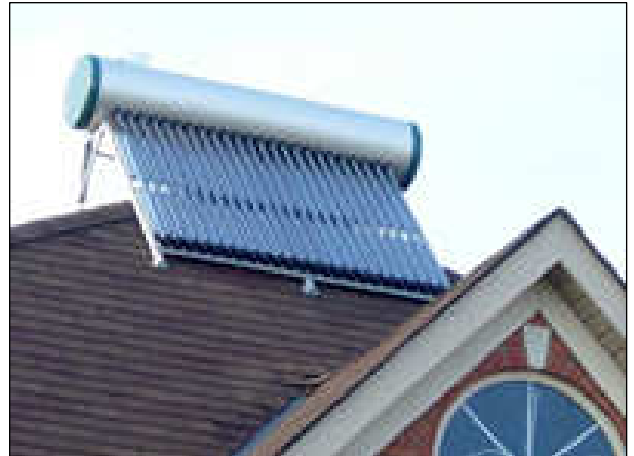
IP-195 Solar Hot Water Unit
